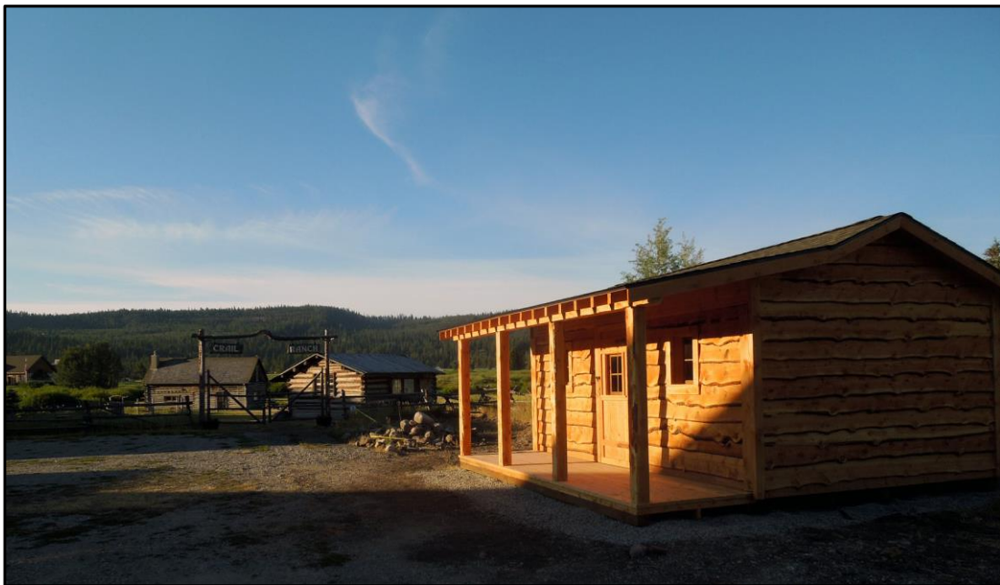
New Crail Ranch Museum Project Center in place late July 2014
